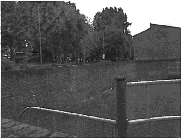
Image 2: View from SE looking towards N.E
